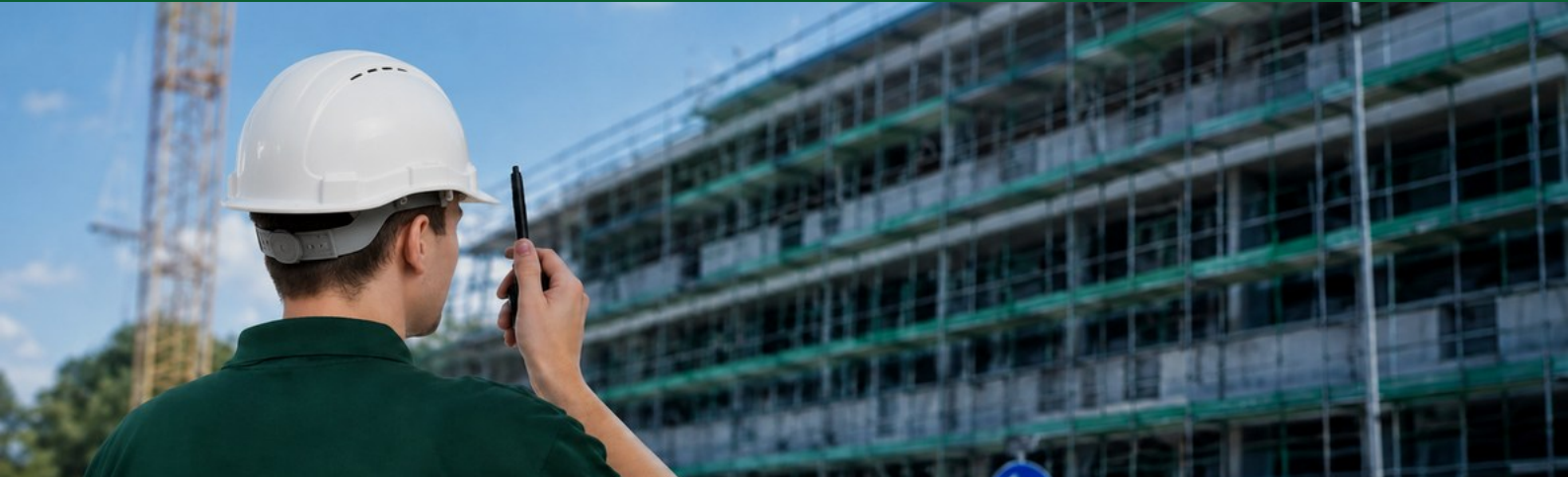
EUROCS safety staff during construction site inspection – fire protection, occupational safety, prevention service
